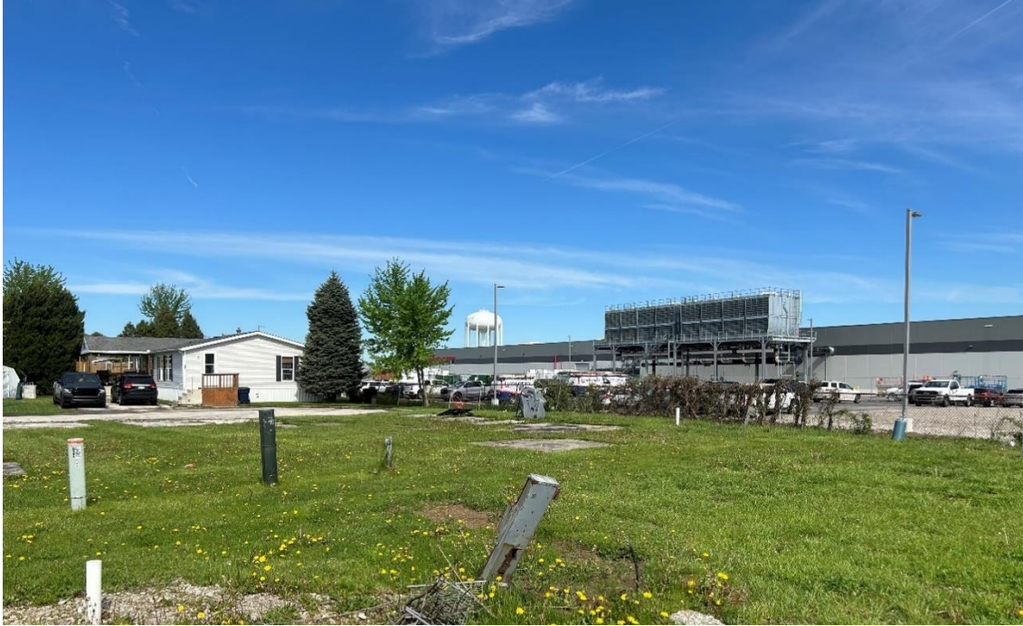
Figure 4: R&D Facility under construction seen from the vantage point of the Friendly Village Estate, 2024. Source: Authors
