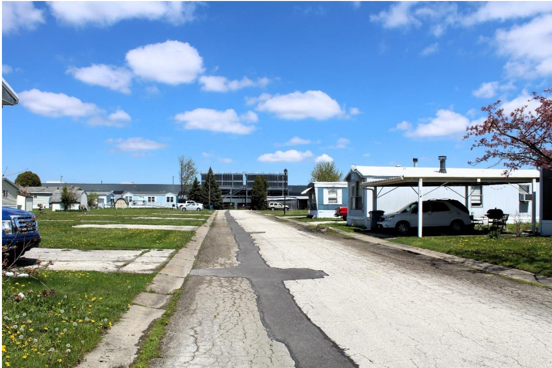
Figure 5: R&D Facility under construction seen from another vantage point in the Friendly Village Estate, 2024. Source: authors
