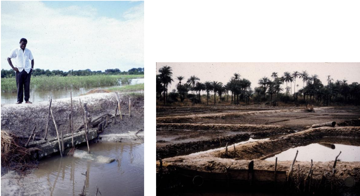
Figure 4. Left: Palm trunk set in main embankment as sluice for water control. Note the difference in water level between polder and waterway. Right: trunk sluice being replaced between individual rice parcels in the dry season. Casamance, Senegal, 1999. Source: Judith Carney
