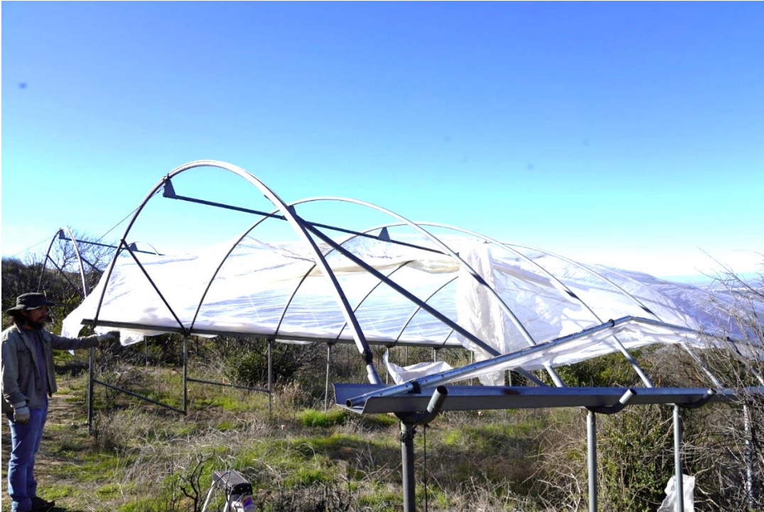
Figure 9: Damaged shelter. Photograph by Author
