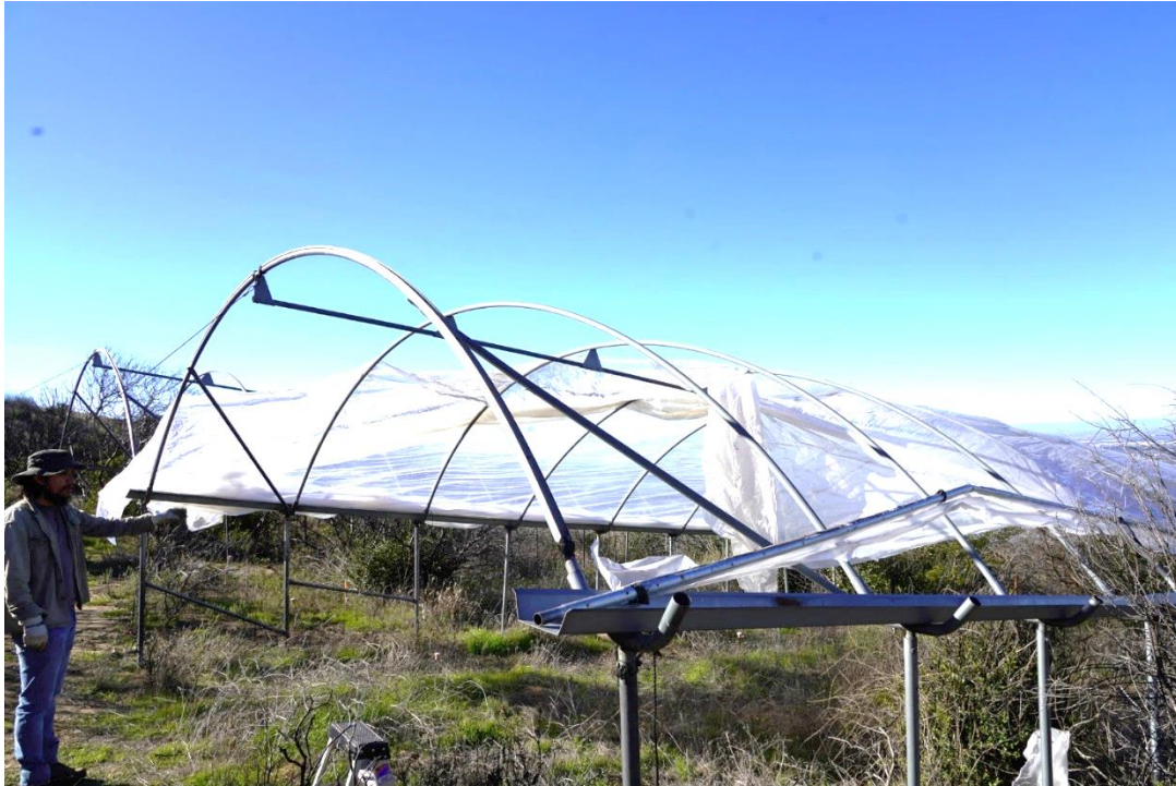
Figure 9: Damaged shelter. Photograph by Author
