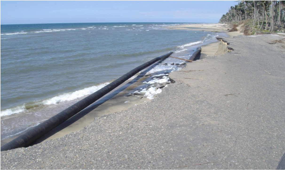
Figure 4: Coastal erosion impacts roads and oil infrastructure in the study sites.
