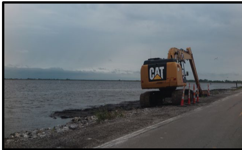
Figure 5: Construction of fishing piers on Island Road, 2020. Photo by Author
