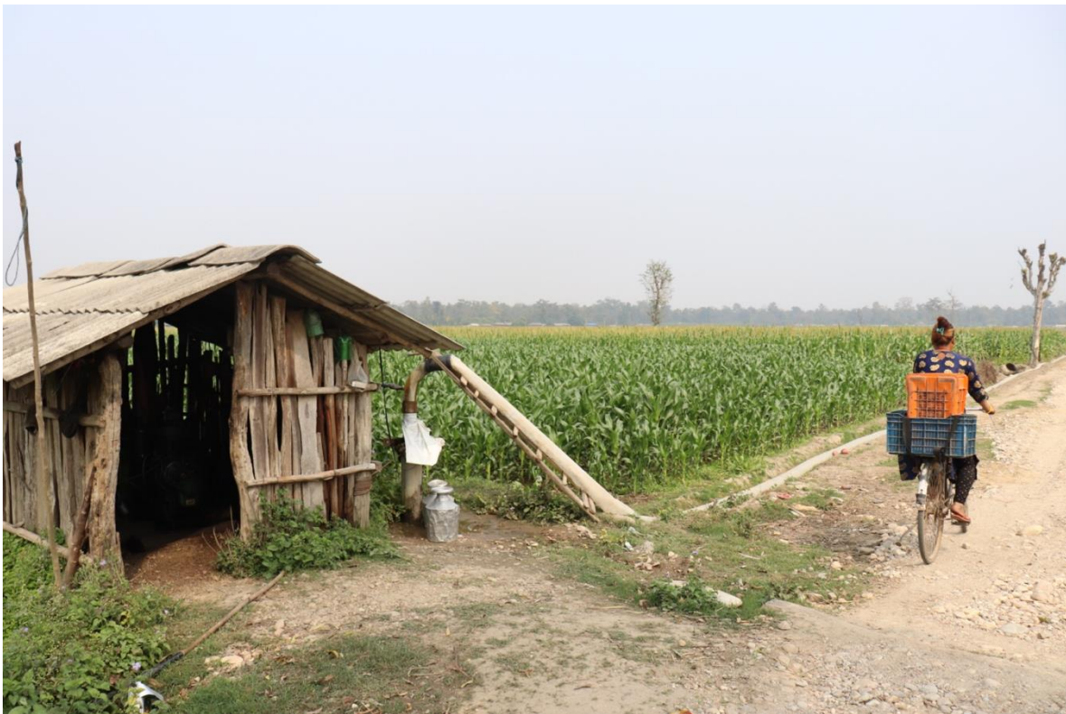
Figure 4: Pump and line as part of village irrigation system. Source: Authors, 2020
