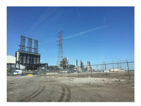
Figure 5: One of the main fixtures of BP's tar sands renovation is the coking tower, pictured on the left.
