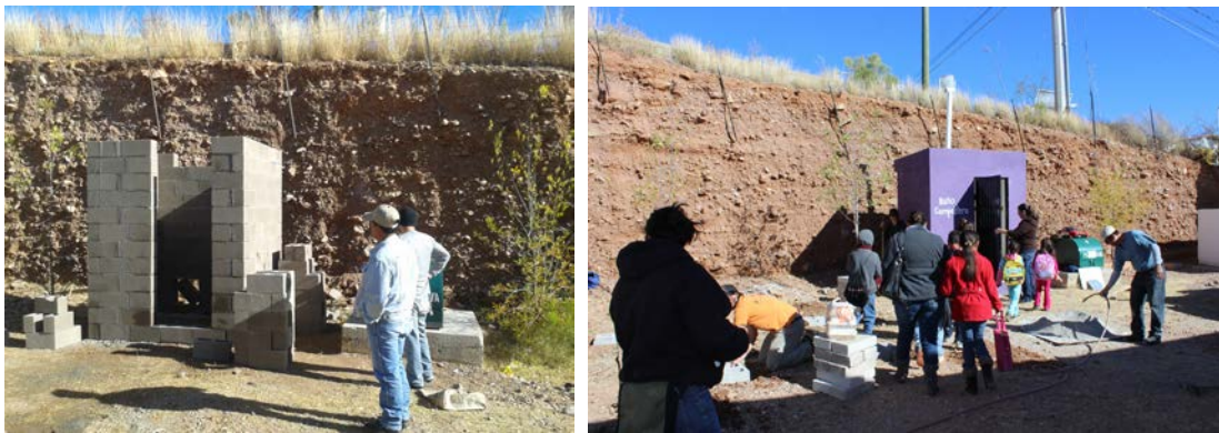
Figure 5. Construction stages of the composting toilet in Nogales. Source: Sarah Kelly-Richards.
