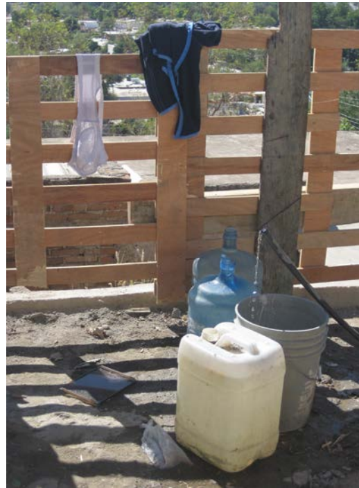
Figure 2. A hose running up the alleyway in a barrio Viejo of Hermosillo serves as informal water pipe. Source: Lucero Radonic.
