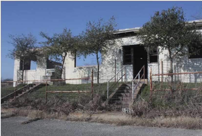
Fig. 2 Exterior of administrative building
