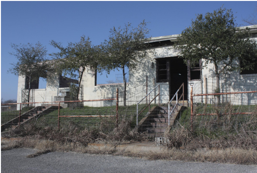
Fig. 2 Exterior of administrative building
