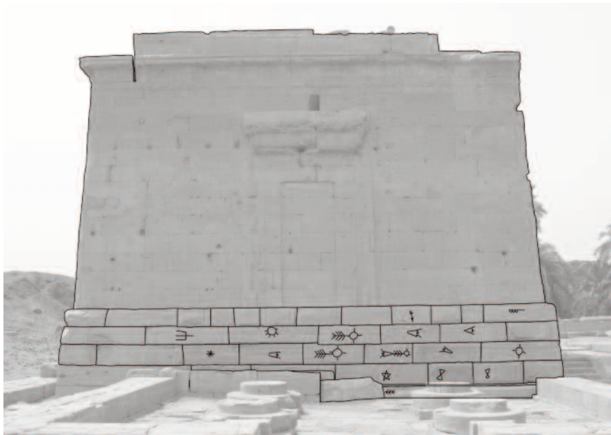
FIGURE 7: A: Eastern exterior wall of the Temple of Isis. The rough, undressed blocks are outlined, and quarry marks accentuated. B: Facsimile detail of the marks.
