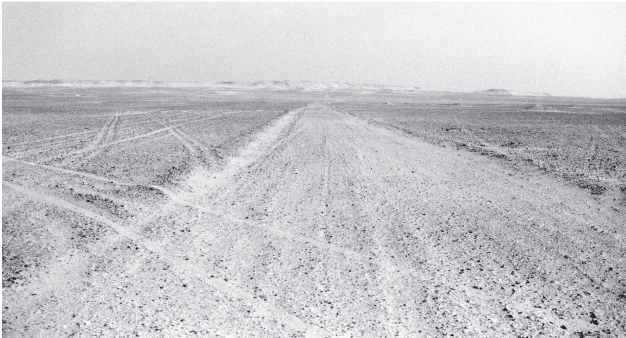
Figure 33: A modern track leading through the desert between Dahshur and Saqqara. The surface is smoothed; irregularities and depressions are leveled to create a plain surface. The residual material is piled alongside the track, so that it is visible over long distances. Tracks in ancient Egypt may have had a similar appearance. (photograph by H. Köpp-Junk).
