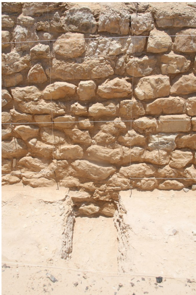
Figure 10: Detail view of the rough limestone masonry in the western “bastion” with a test trench exposing the two foundation courses (Photograph: P. Carstens)
