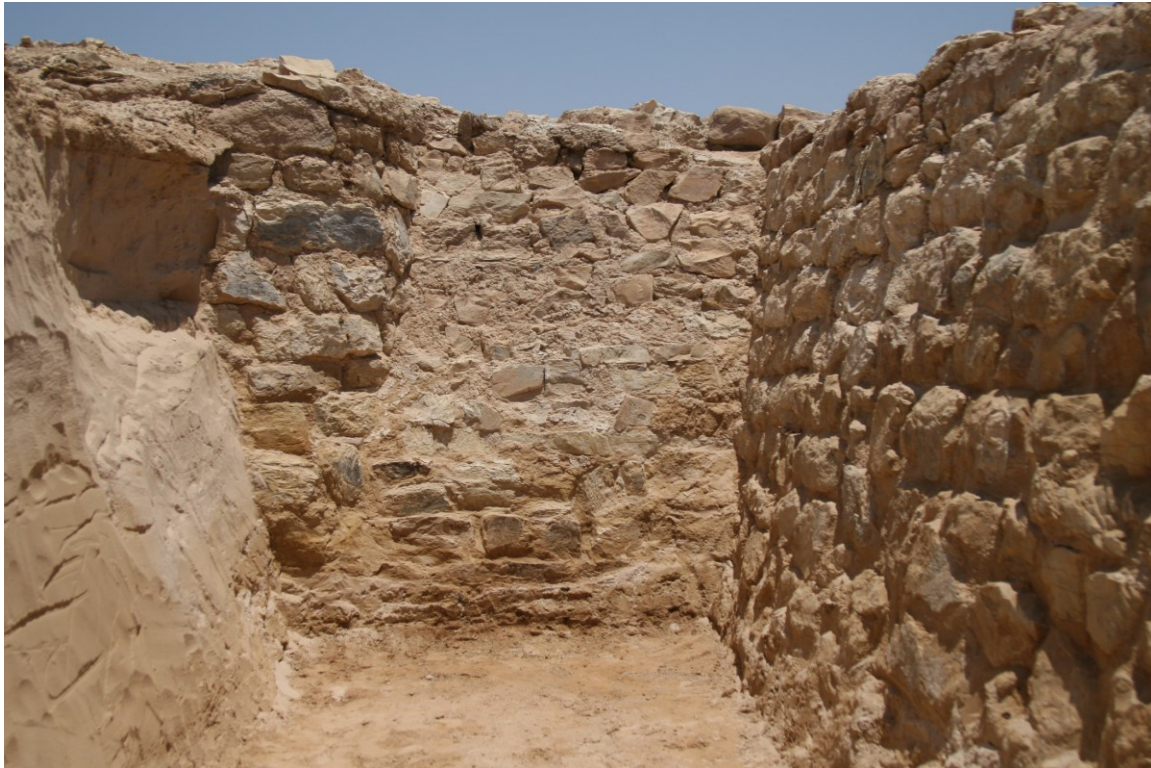
Figure 13: Detail view of the blocked-up western entry to the fort (Photograph: P. Carstens)
