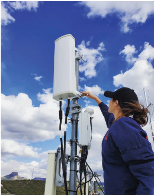
Ms. Blackwater installing broadband internet at Diné College
