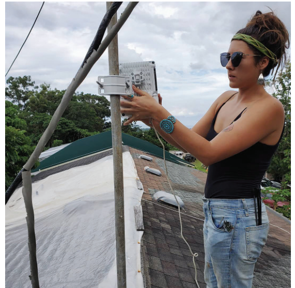
Ms. Blackwater installing broadband internet in Hawai'i
