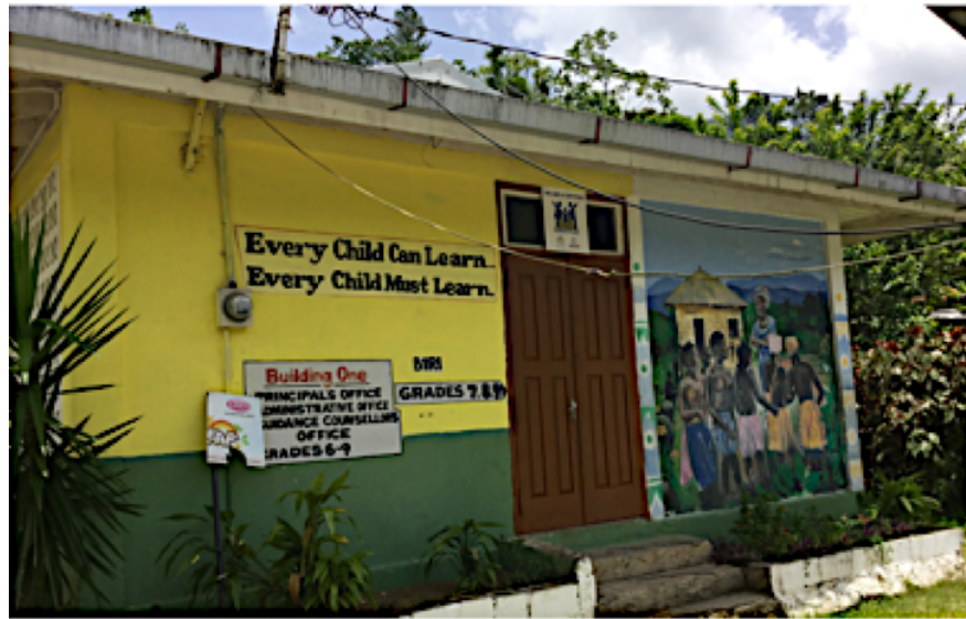
Figure 11. Mooretown Elementary School (photo CMB)
